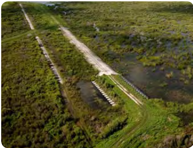
Delivering essential restoration benefits to America's Everglades. (Photo by Mark Bias)
